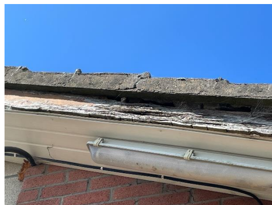
Plate 3-2 Gaps in fascia board
